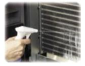
Disinfect and deodorize the evaporator coil and drain pan with SANI C-N-D<sup>TM</sup>, an EPA registered biocide, fungicide, viricide, and mildewstat. The broad spectrum biocide in SANI C-N-D<sup>TM</sup> assures control of many airborne pathogens that can be spread via contaminated air handling equipment.
